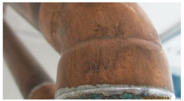
Above: DWV (drain-waste-vent) fitting improperly used in a riser where it was subjected to pressure for which it was not designed for.
