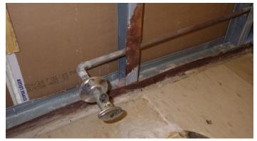
Above: Copper pipe in direct physical contact with aluminum framing causing galvanic corrosion. In this example, it was the frame that corroded.
