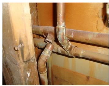
Above: Substandard solder connection with no solder on the contact surfaces creating a snug-fir connection.
