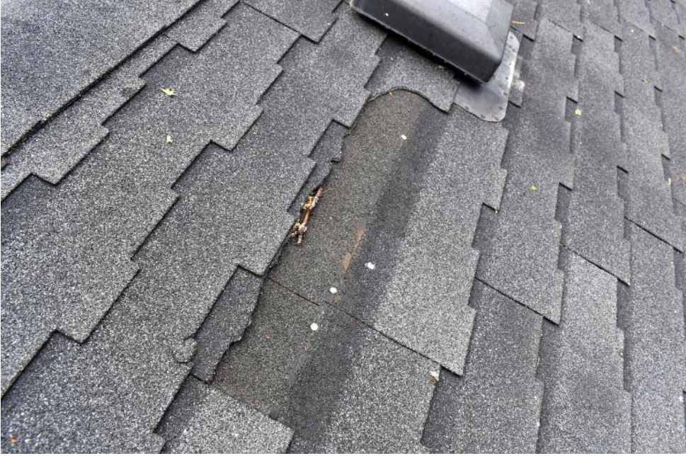
Figure 2 – Shingles are not structural elements. The repair does not involve a structural engineer, but the cause of roofing damage may be assessed by a building envelope investigation.
