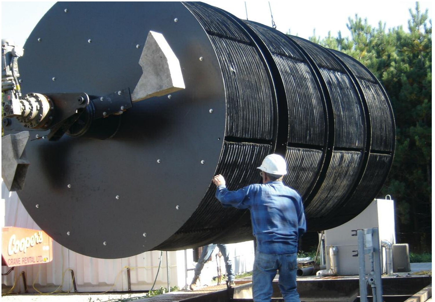
Photo credit: RBC, Rogers Pass, BC https://napier-reid.com/products/bio-rotortm-rotating-biological-contactor-rbc/ (DSC04498 - 6-Mono-Mills)
