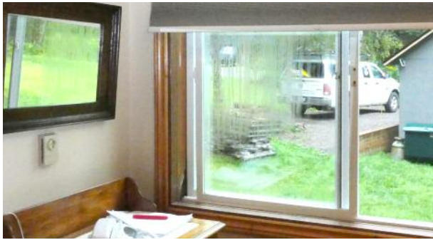
Figure 6. Moisture damage of the window's jamb due to condensation, related to a poor installation. Note the condensate on the window.
