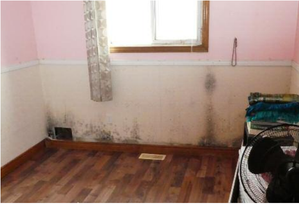
Figure 5. Staining along base of wall was consistent with air leakage.
