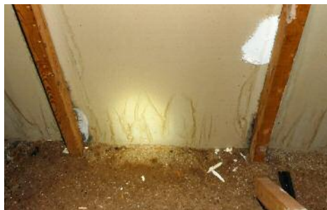
Figure 10. Water stains caused by thawing frost that dripped, which had formed on roofing nail tips due to condensation.
