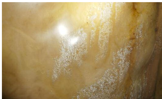
Figure 2. Condensation observed on polyethylene vapour retarder.
