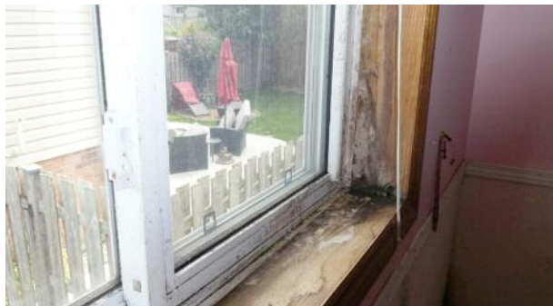
Figure 7. Moisture damage of the window's jamb and sill due to condensation, related to a poor installation.
