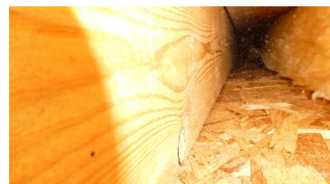
Figure 4. Interior view of wall stud cavity revealed a void in insulation. This 'thermal bridging' contributed to wall staining.
