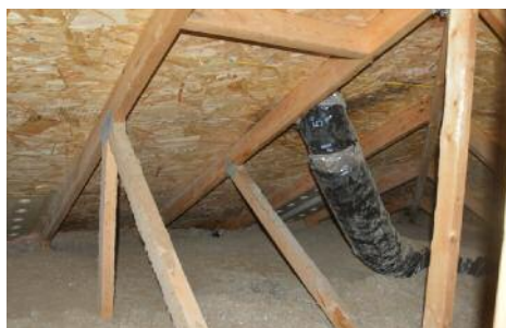
Figure 13. Local moisture damage to wood roof sheathing due to a small air leak in a bathroom extraction fan vent.
