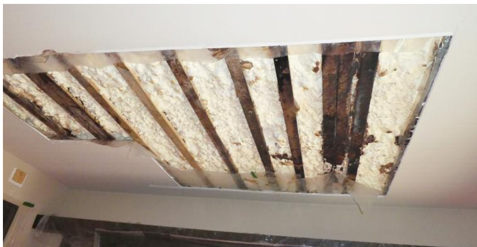
Figure 14. Rotted wood roof joists.
