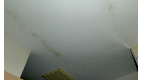
Figure 8. Staining on bathroom ceiling.
