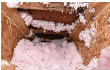
Figure 11. Poor airflow through the flat roof's attic space contributed to condensation, which caused wood rot of the structure.
