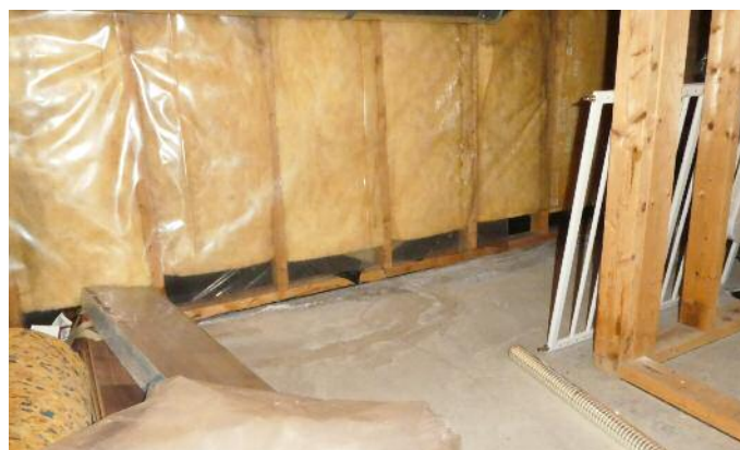
Figure 1. Staining on basement floor slab resembles foundation leakage. In reality, staining was due to condensation from discontinuity in insulation and vapour retarder.
