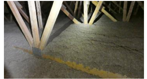
Figure 9. Lack of attic insulation. The roof rafters were inline with the interior ceiling stains.
