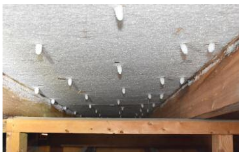
Figure 12. Frost formation within an attic. A disconnected supply air duct introduced warm humid air into the cold space.
